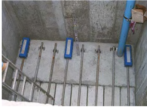
Concrete Block Underdrain
